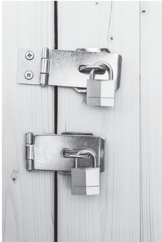
Incorrect and correct mounting of a latch. Forgot your keys? No worries, just remove a few screws instead.
