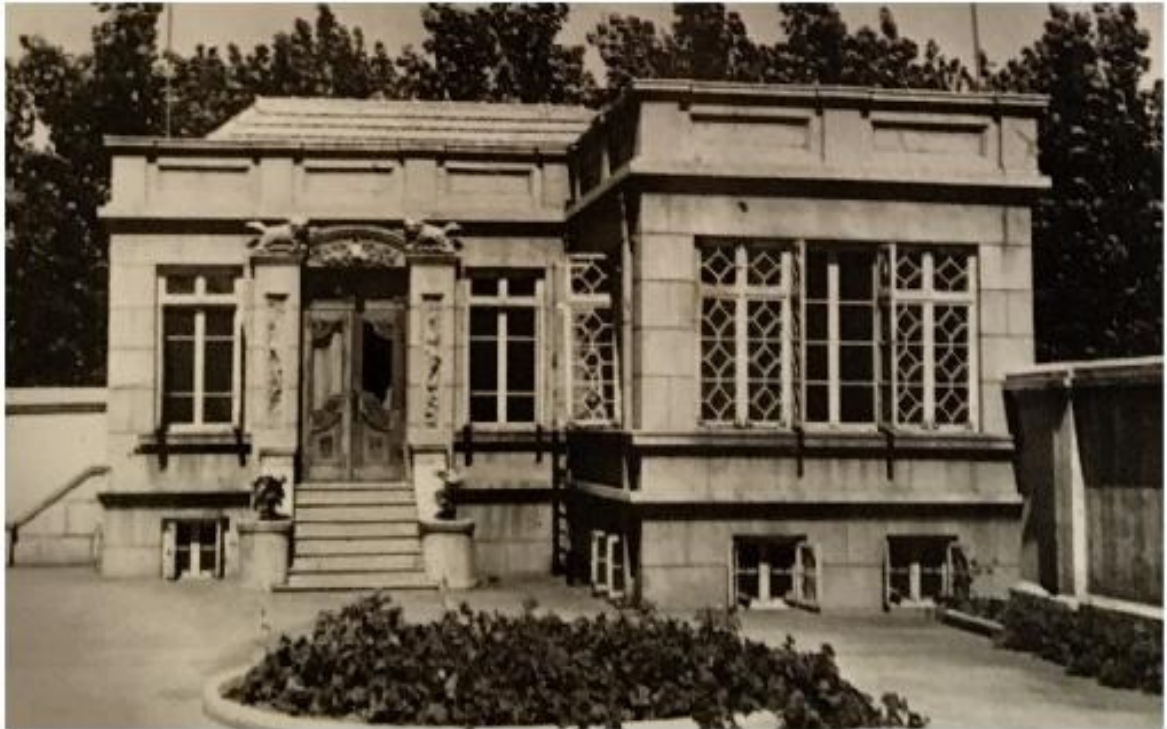
The house in Mukden. The bamboo poles holding up the aerial for her transmitter can be seen at either end of the roof.
