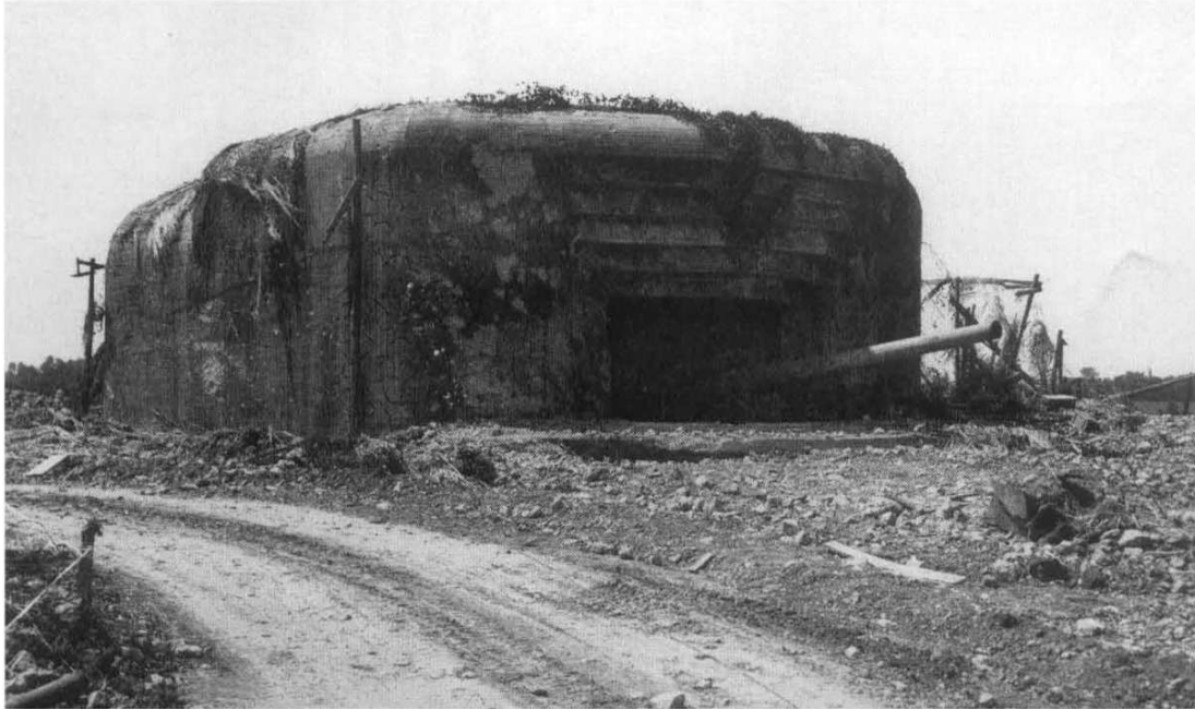
The Germans poured millions of tons of concrete into the Atlantic Wall. This fortified position, at St.-Marcouf behind Utah Beach, had steel-reinforced concrete walls thirteen feet thick. Despite furious air and naval attacks it was still firing on D-Day plus two. (U.S COAST GUARD)
