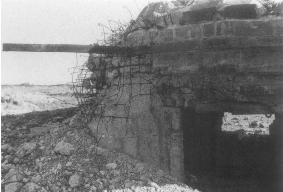
A badly damaged German fortification at Omaha Beach, showing the extent of the steel reinforcing rods and the thickness of the concrete. This fortification looked down on Easy Red sector and had a 75mm cannon that fired through the morning. It was finally put out of action by infantry tossing grenades into it. (U.S. ARMY SIGNAL CORPS)
