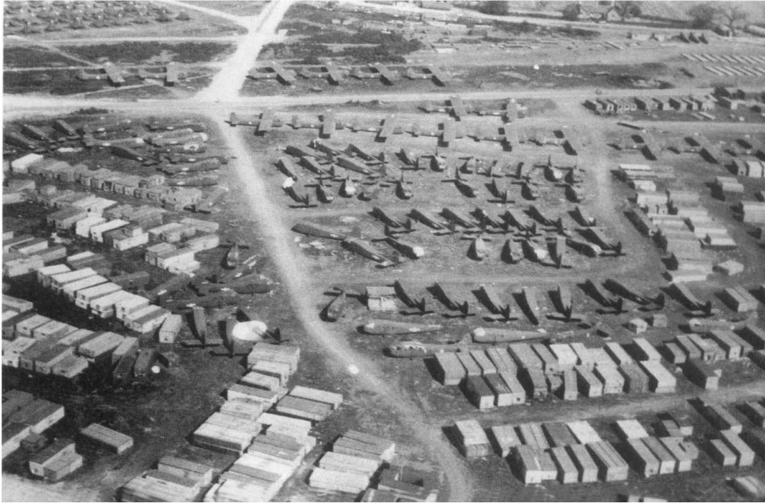
There were other production miracles. Here U.S. Army Air Force gliders arrive in England crated in parts (foreground), are uncrated and have their fuselages put together (center), and have their wings attached (top) to complete the assembly. (WIDE WORLD)
