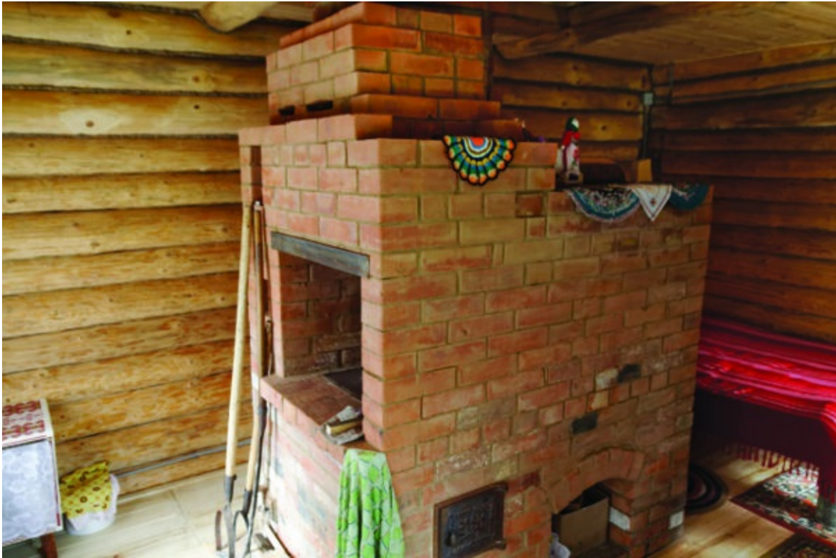
Figure 3.30. A great oven used for malt drying. Kshaushi, Chuvashia, Russia.
