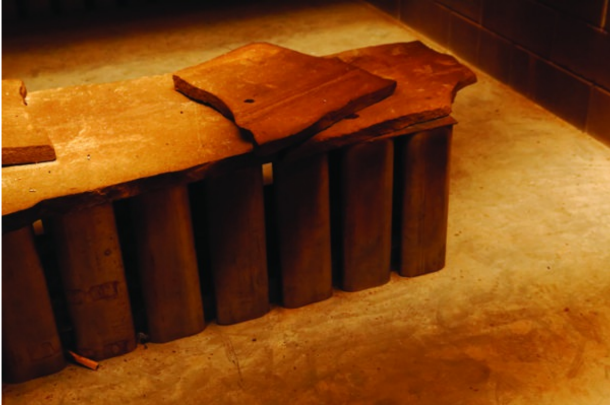
Figure 3.25. Kjerringa visible inside a sâinn with the planking removed. Tautra, near Stjørdal, Norway.
