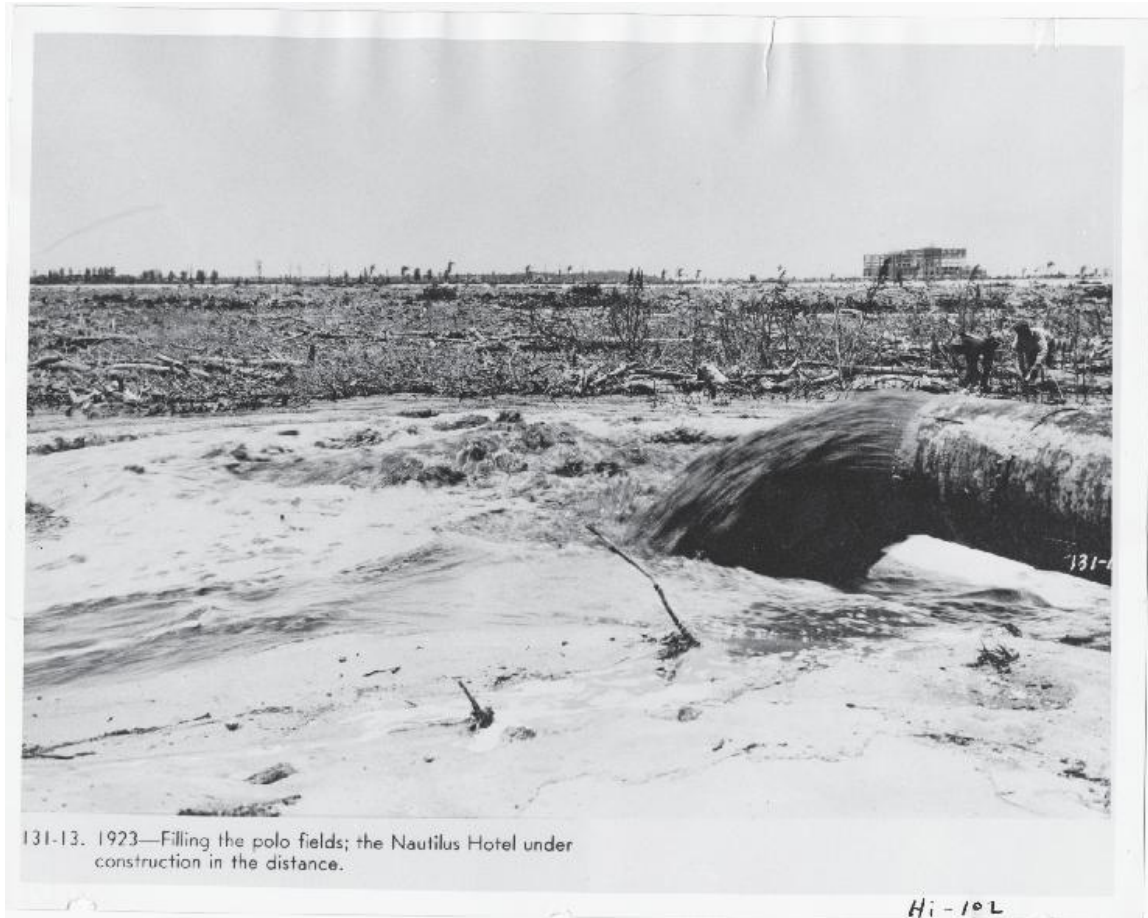
Dredger pumping "soup" up from the Biscayne Bay to make more room for development on Miami Beach. (Photo courtesy of Miami Beach Digital Archives)
